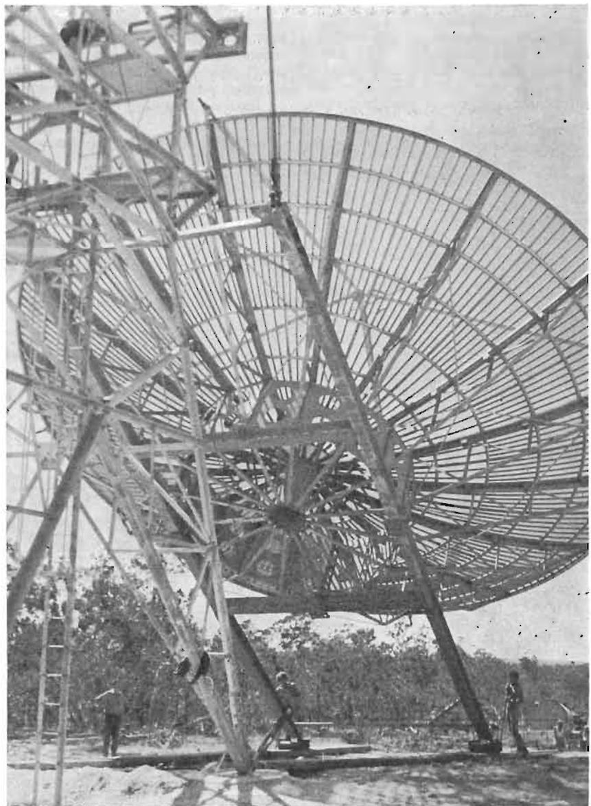
Fig. 12 — Lifting 12m Dish at Munmalary.
