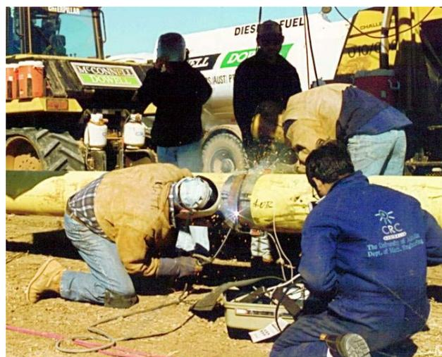
Any person or company interested in the detailed results of the research work should contact the CRC for Welded Structures to inquire about participation in the on-going research work and thereby obtain the outcomes and conclusions of the work done so far on welding X80 thin-walled pipe.
